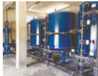
Surface Piped (package piped) filtration systems with Epoxy coated St-37 tanks
